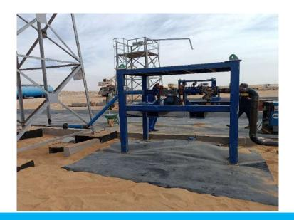
•Inlet and outlet meter connection Inlet and outlet of two meters are fabricated and welded.
